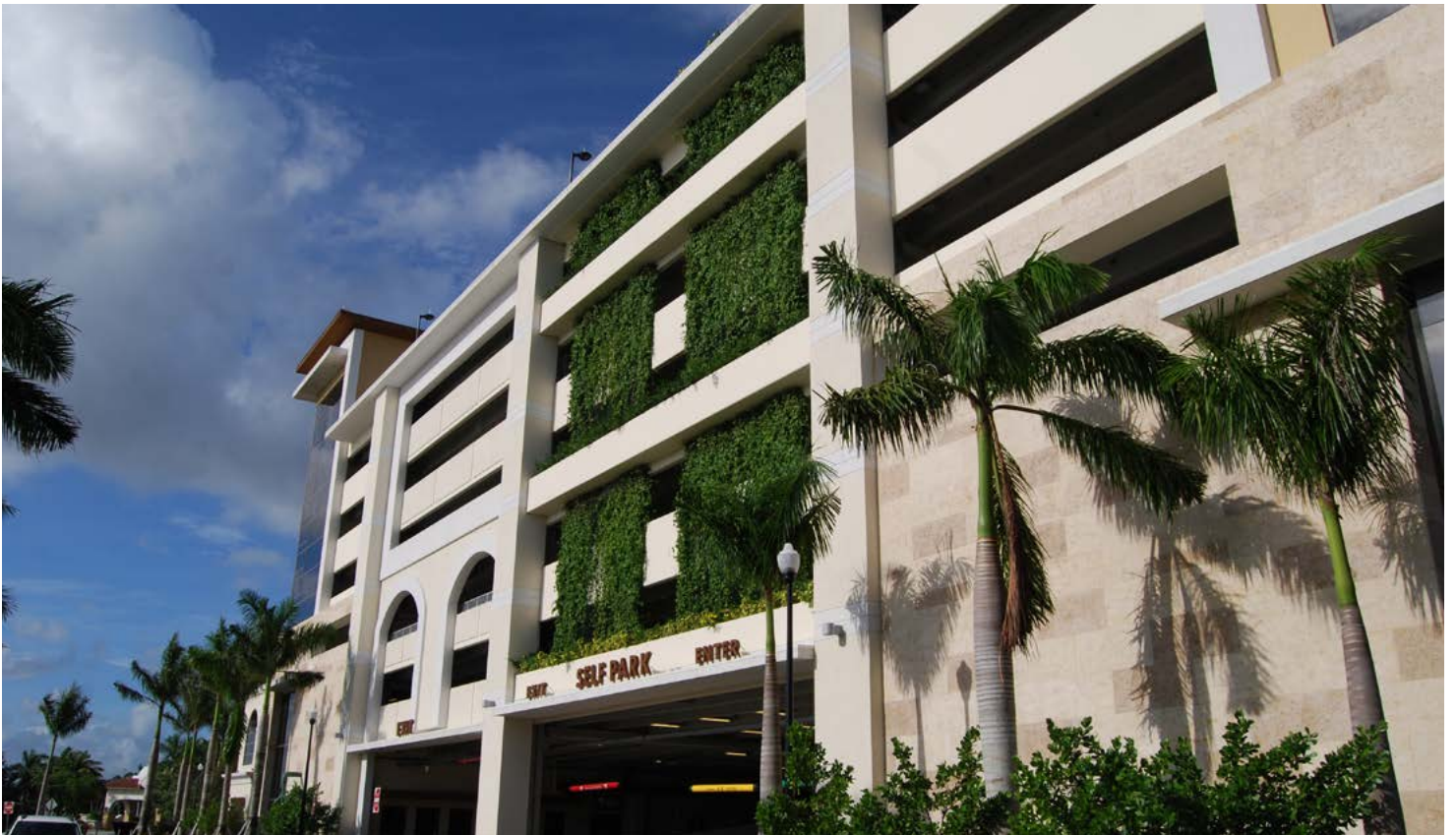
Project: Seminole Casino Coconut Creek, FL • Architect: Friedmutter Group • Contractor: Moss Anderson
