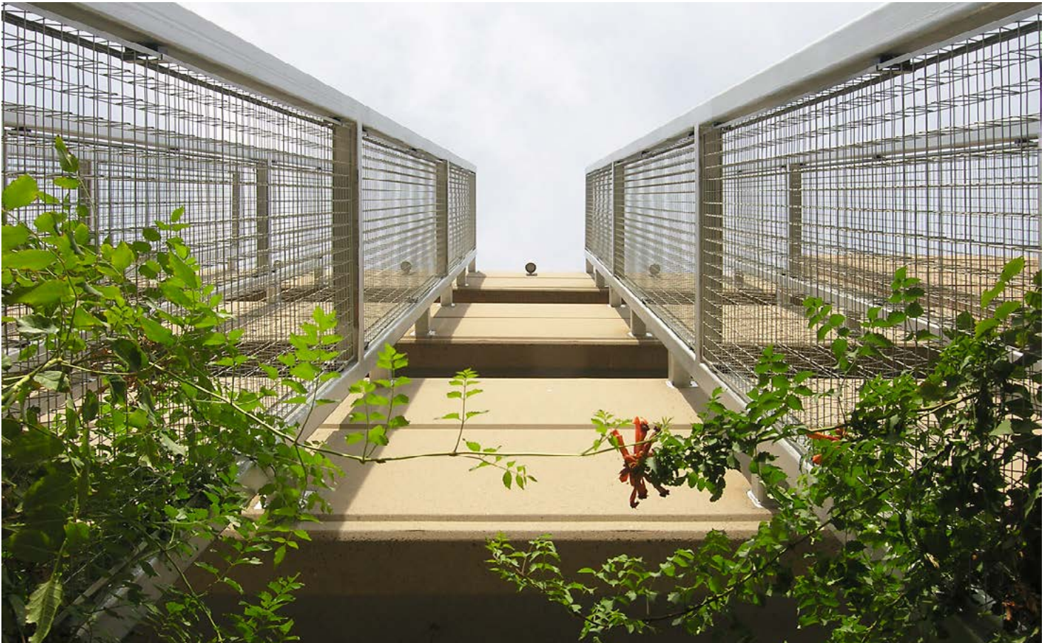
Project: LDS Institute at Arizona State University Parking, Tempe, AZ • Architect: Architekton • Installer: Skyline Steel • GC: Layton Construction
